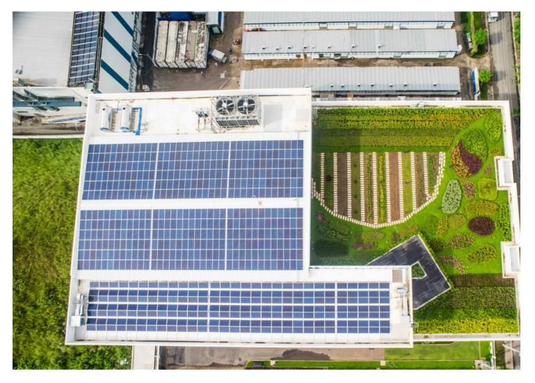
Solar panels on a roof at Deutsche BekleidungsWerke in southern Vietnam. The 18,000 square metre facility opened in November this year and is equipped with solar panels to provide up to 20 per cent of the energy required for operations during the droughts experienced in the dry season.
